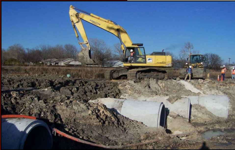
Road construction to improve drainage to Business 79 in Taylor, Pct 4.
